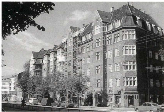
Åhusene, Åboulevard 12–18, Kbh. Ulrik Plesner 1895–98.
