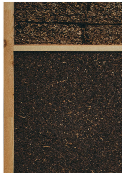
A view of the exterior panel (bark & pine cones) and leaf insulation. (Top exterior panel removed for view)
