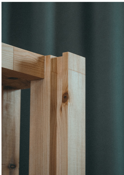
Grooves in the studs where the composite panels can be inserted into.
