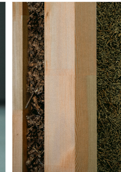
A close up, showcasing the fit of the panel and insulation block in the wall frame.
