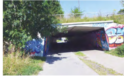
Figures 5 and 6. The tunnel before and after
